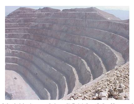
Figure 7. View of a benched slope in an open pit mine used to illustrate the application of the proposed stability analysis tools.
